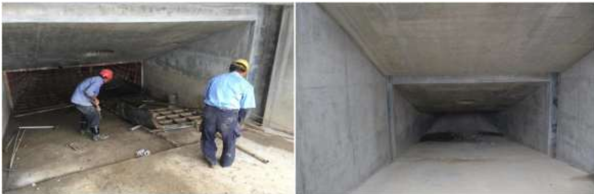
Figure 5.4-1 Demolition of steel formwork, Figure 5.4-2 Effect after removal
