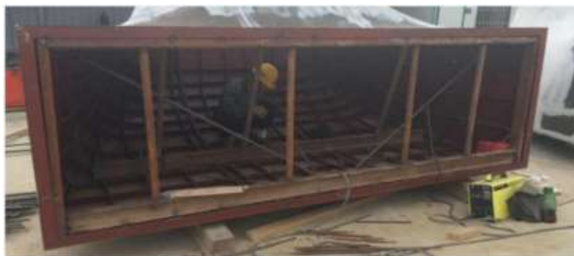
Figure 5.3.2-1 Reinforcement process at the inlet of the flow channel
