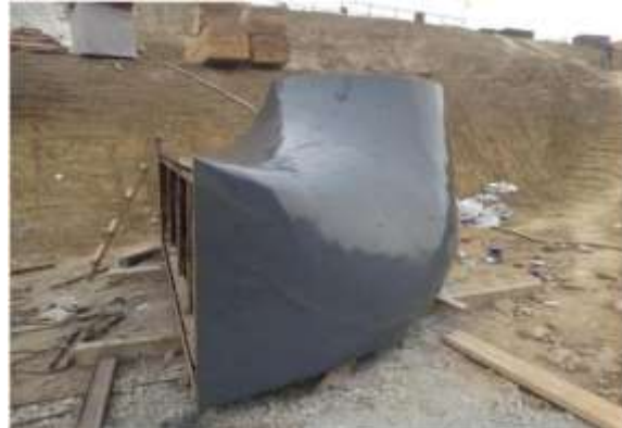
Figure 5.2.4 Surface treatment of the steel plate
