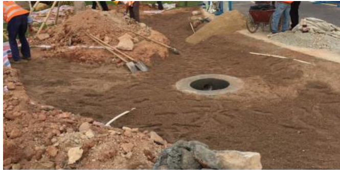
Fig. 1.7 Active Composite Soil Paving
