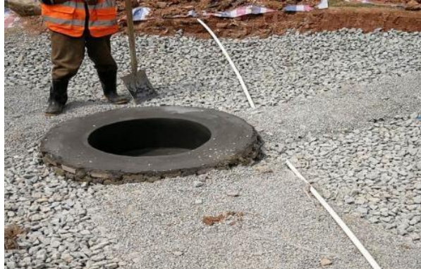
Fig. 1.5 Masonry of overflow well
