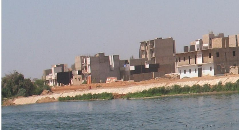
Photo 1: ORYX lake with one of its parts backfilled and intended for housing
