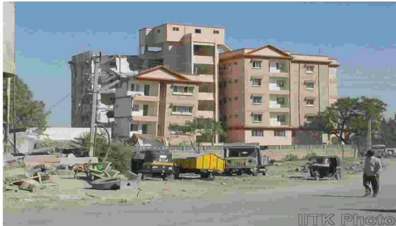
Fig. 2 Failure of OGS building during Bhuj earthquake.
